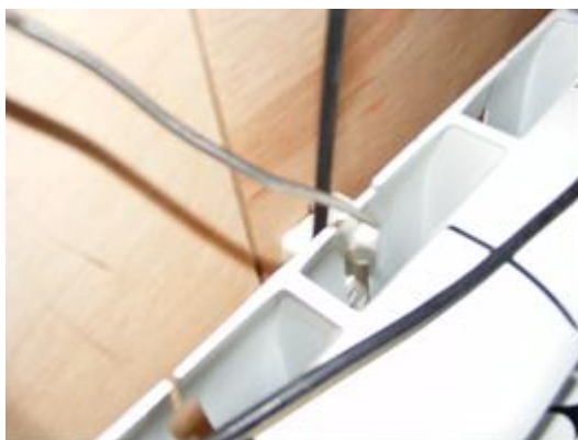
Figure 3 Detail of “air off” probe and oil probe connection
