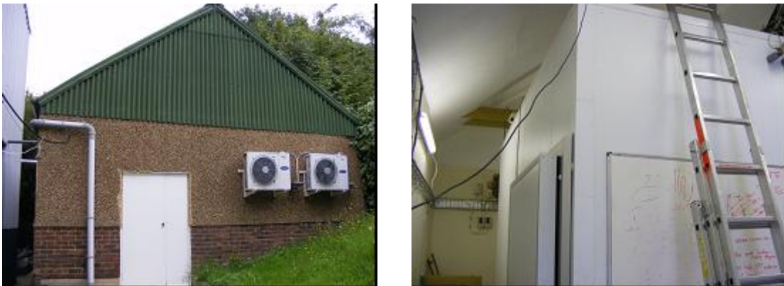
Figure 1 External and internal chambers at BSRIA
